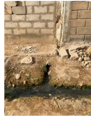
Self-dug drainage system and connection to dwelling.
