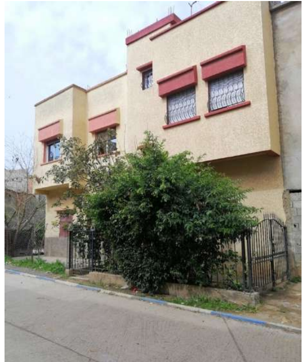
[Fig.8] Plots Housing lots for new residents (outside of the douars) « from the author », 2021.
