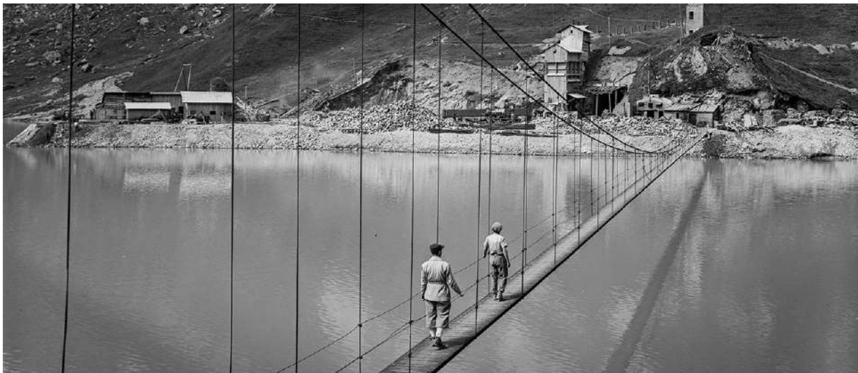
[fig.2] Morasco dam construction process. Source: ENEL
