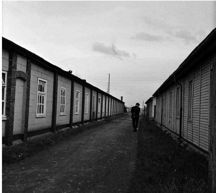
[fig. 5] Tenements in Durisol blocks and wood in the mining settlement of Zwartberg. Source: Geheugen van Genk.
