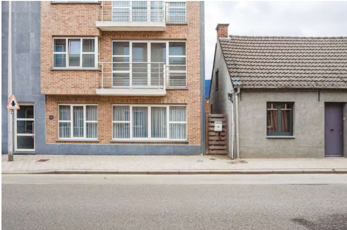
[fig.1] Zoom on the architecture of the ongoing village transformations in Kessel, Nijlen where new apartment buildings are nested next to old farmhouses. Source: BKP Nijlen, PLUSOFFICE, 2017, image by Pieter Vandenhoudt.
