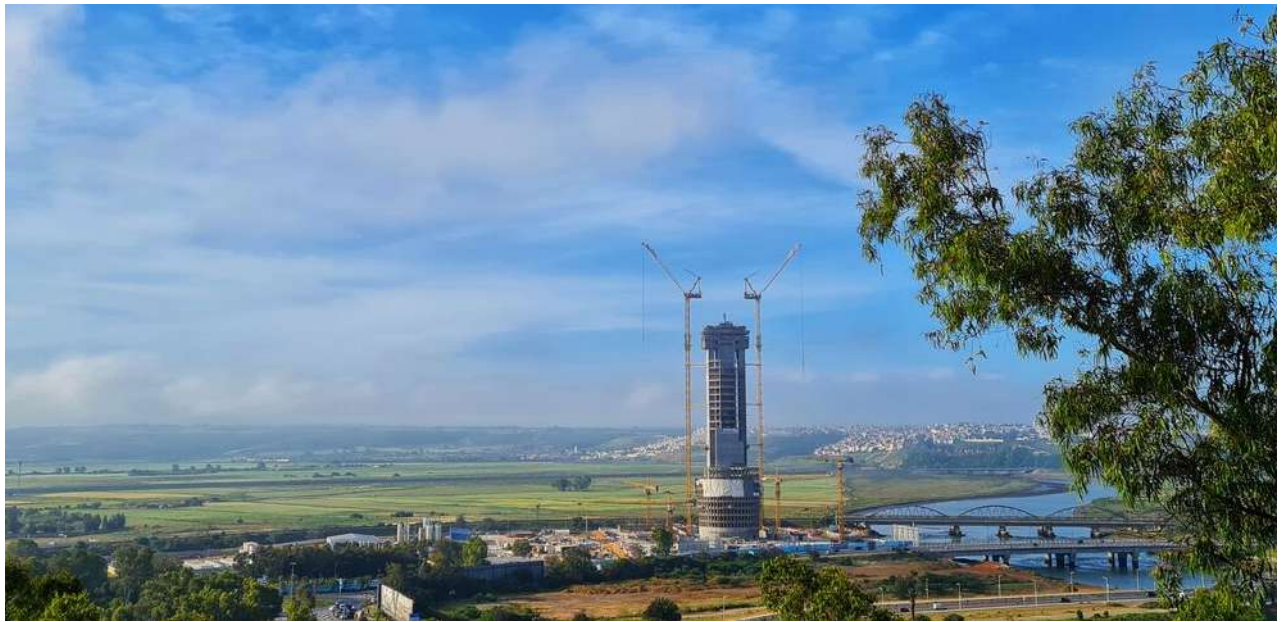
[Fig.1] Mohamed VI tower, the tallest tower in Africa, from « Besix.com ».
