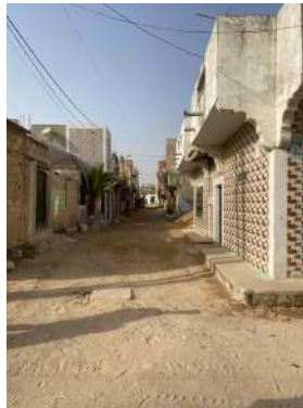
Street with underground drainage installed by residents of one sector.
