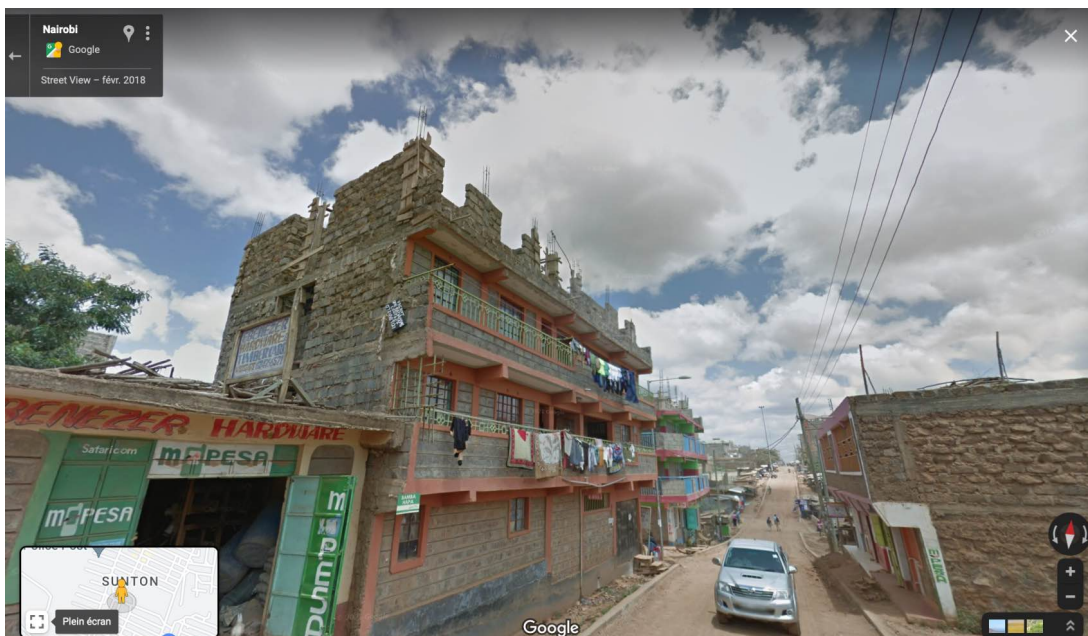
Figure A1: An unfinished building
