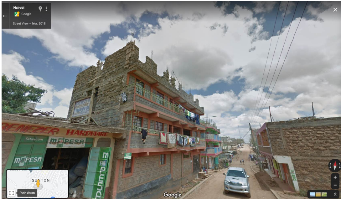
Figure A1: An unfinished building
