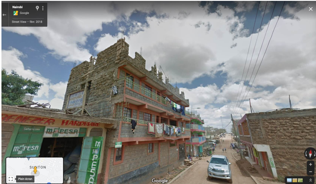
Figure A1: An unfinished building
