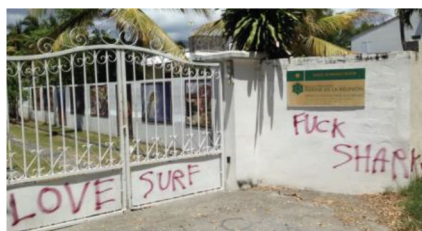
Fig. 4 Deterioration at the entrance to the RNMR premises (December 4, 2018)
