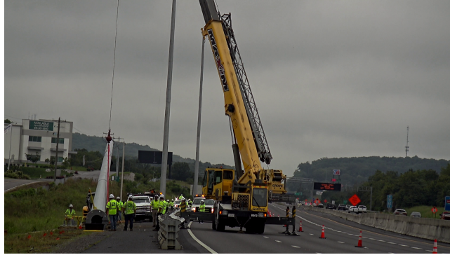
Fig. 1: Installation of a roadside pole on the I-24
