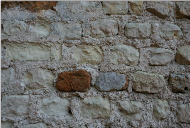
Fig. VIII.4.10 - Aspect non lissé des joints 30001 © Cliché A. Remy.
