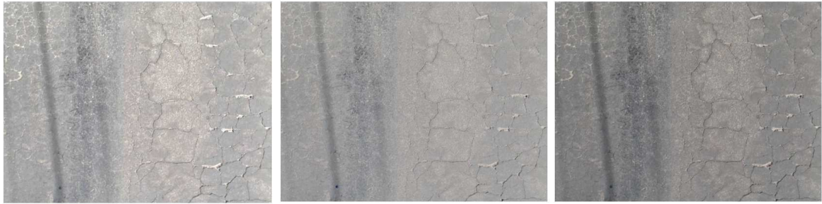
398 399 Figure 9. Example of an augmentation where the lighting was artificially changed, (middle image is the 400 original one)
