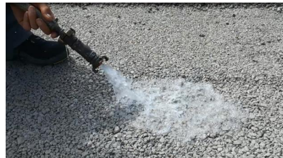
Figure 6 : In situ placing of the excavatable porous cement treated aggregate and visual observation of it high draining capacity
