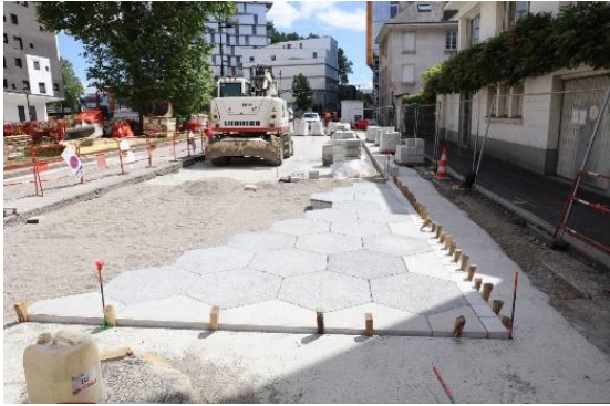
Figure 17 : (Left) Insertion of the slab along the block line. (Right) Encapsulation of a network access. The concrete blocks ensure the removability of the slabs around the access
