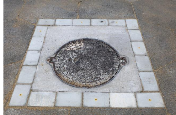
Figure 17 : (Left) Insertion of the slab along the block line. (Right) Encapsulation of a network access. The concrete blocks ensure the removability of the slabs around the access
