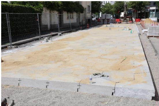
Figure 18 : (Left) Joint filling with 0/2 mm sand before the casting of surrounding concrete edge beams to confine the slab movements. (Right) Final aspect of the demonstrator
