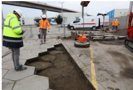
Figure 3 : Assembly-dismantling of the RUP with interlocked slabs.
