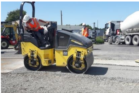
Figure 6 : In situ placing of the excavatable porous cement treated aggregate and visual observation of it high draining capacity
