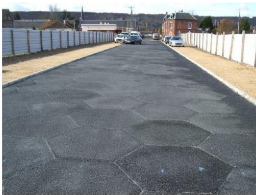
Figure 1: First RUP prototype with independent slabs, Saint Aubin les Elbeufs, 2007
