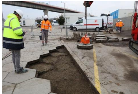
Figure 3 : Assembly-dismantling of the RUP with interlocked slabs.
