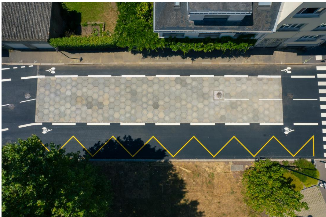
Figure 19 : Drone overview of the finalized RUP-FS demonstrator (Credits Eiffage Route)
