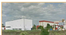
Source: CEREMA Zone Industrielle de la route des Varennes: Azelis-Peroxides, Bioxal, ALEM, Technic.
