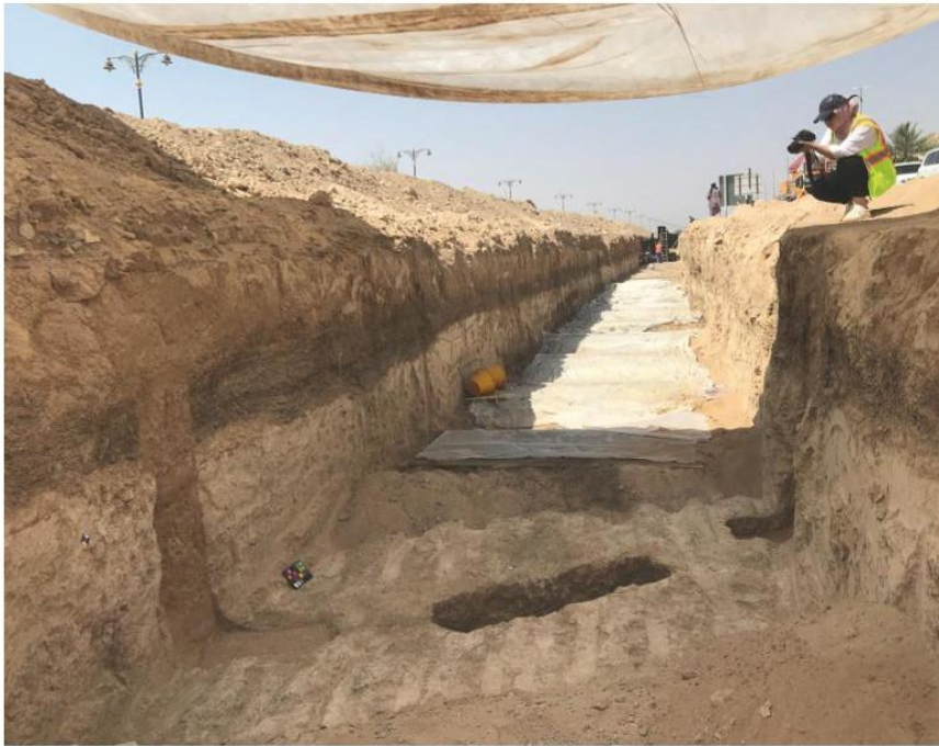
FIGURE 9. Zone C showing three consecutive falaj thuqb (one in plan and one in each section) crossing the line of the border fence trench in Zone C.
