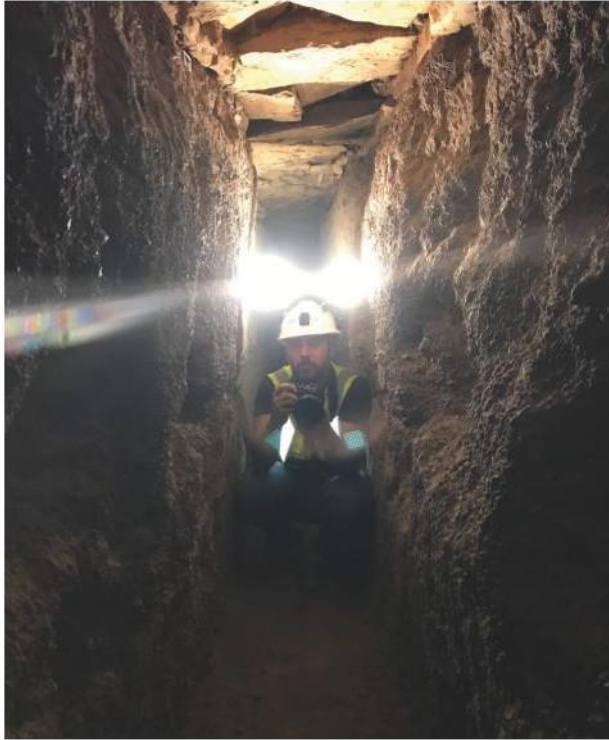
FIGURE 5. 3D scanning and photogrammetry in progress inside the historic Jīmī falaj.
