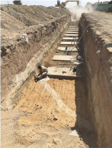
FIGURE 2. View looking south along the border fence in Zone Ab showing the sequence of works, with archaeological investigations and recording of a falaj in the foreground, and in the distance backfilling around the fence foundations.
