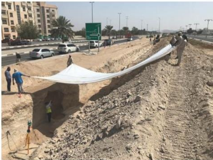
FIGURE 4. Photogrammetry in progress in Zone C.
