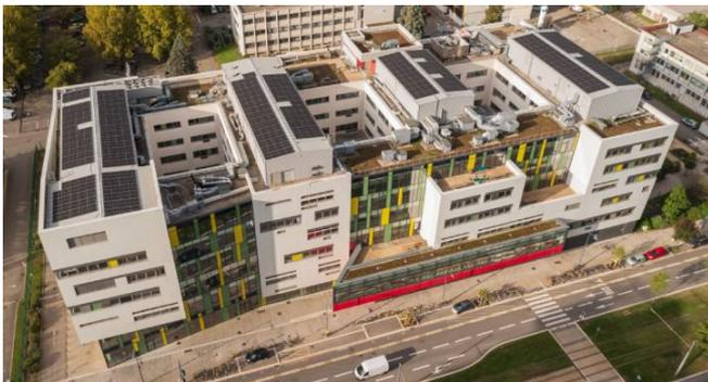
Fig. 2. GreEn-ER building with 183kWp PV panels
