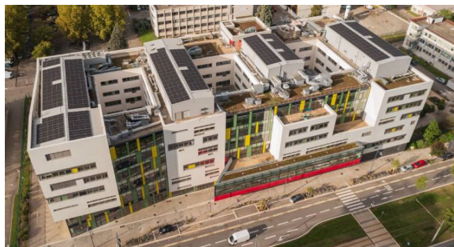
Fig. 2. GreEn-ER building with 183kWp PV panels
