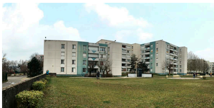
Figure 3. Overview of the social housing complex used to illustrate the methodology [24].
