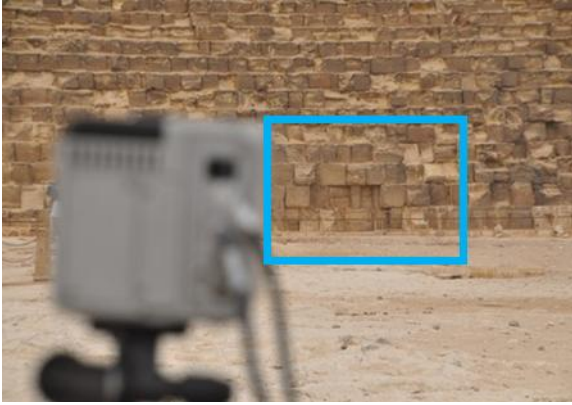
Position of the microbolometer camera 50m from the East face. The anomaly detected is inside the blue rectangle.
