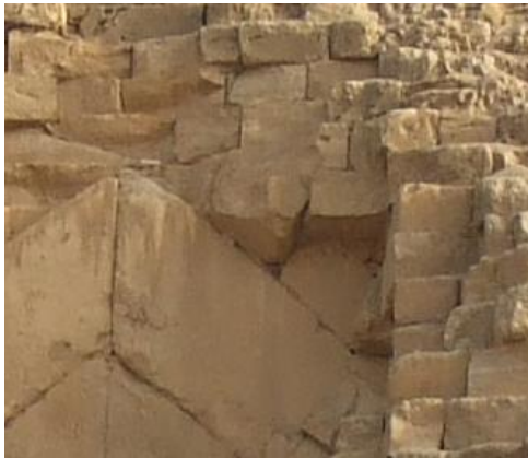
The blocks are fitted directly on the top of the top right rafter.
