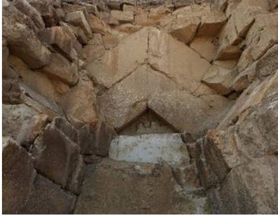
Close-up of the rafters at the North face entrance.
