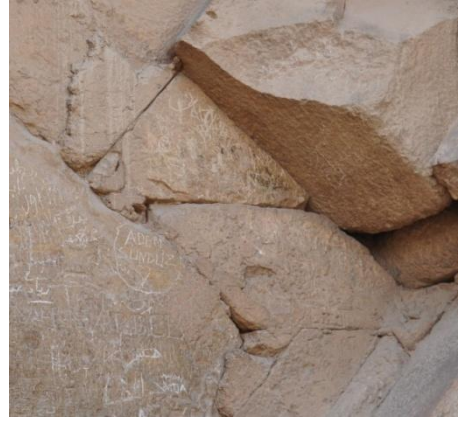
Close-up on the wedging technique: - 2 beveled wedges at the bottom, - a perfectly cut block at the top, - below it, the wedge to receive the temporary wooden shim.
