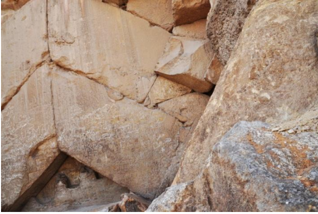
View of the blocking wedges at the foot of the top right rafter: - the lower part is wedged first, using 2 wedges cut at an angle for 2-phase insertion. - a single block is used for the upper part.
