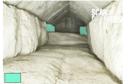
Blocks already in their final positions. These are the blocks laid from the beam across the chamber to the rear of the chamber.
