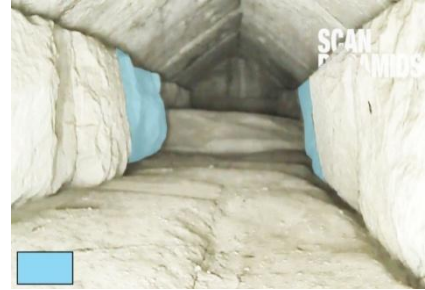
The blocks were stored in the center of the chamber to give the counterweight the necessary length of travel when braking the descent of Strabo's Portcullis.
