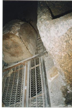
The perfect flatness of two sides of the abandoned block can be seen in this 1998 photo. The block stands on a protective grid covering the digging between the North wall and the sarcophagus.
