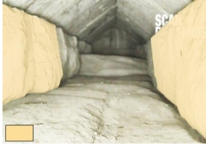
The blocks of the counterweight system. Before the portcullis was lowered, they were pushed back to the level of the beam running through the chamber.
