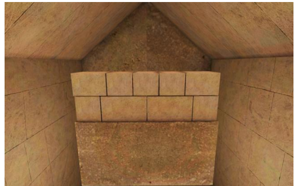
Strabo's Stone in its final position at the front of the second entrance chamber. Additional masonry was built above it. Two blocks of this wall are visible from the outside, above the Strabo Stone and behind the lower pair of rafters.
