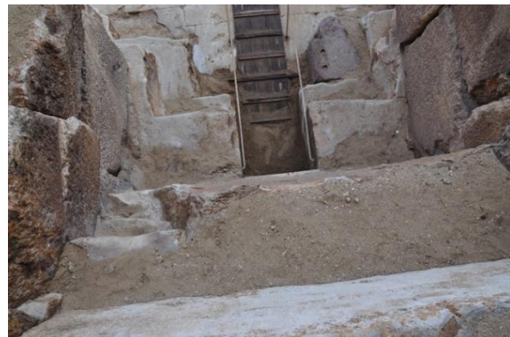
Looking down from the platform in front of the Strabo Stone onto the descending corridor. Lateral benches of 2 cubits each on either side of the descending corridor left a 3-cubit well centered on the 2-cubit-wide corridor. The remaining cubit was distributed on either side of the descending corridor to create supports for closing slabs.
