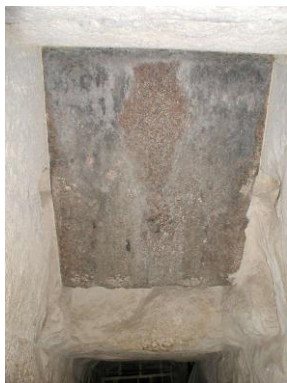
View, from the descending corridor, of the underside of the first plug block thrown into the ascending corridor.
