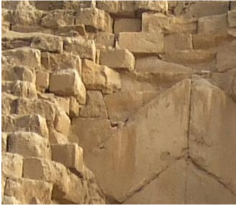
Block layout above the top left rafter
