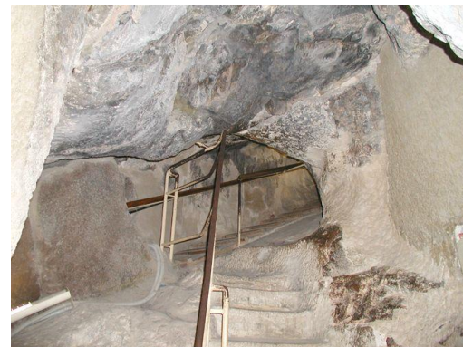
View of the third plug-block, partly broken, upstream of the second, from the al-Ma'mun's tunnel dug by the looters. A well has been dug linking the two corridors.
