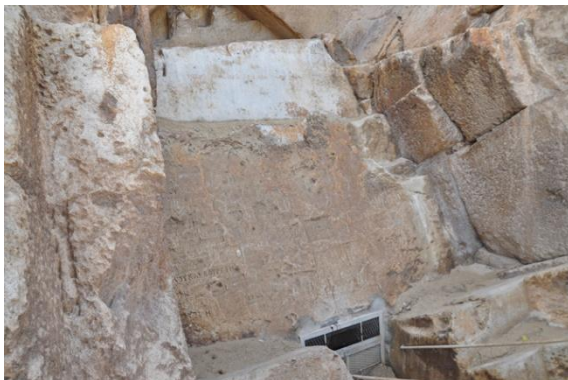
View of the descending corridor, the large oblique slabs and the Strabo Stone. The side walls form part of the basic structure of the first entrance chamber and are 7 cubits (3.68 m) apart.
