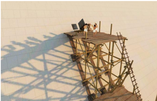
The exterior wooden scaffolding providing access to the pyramid's unique entrance. The Turah limestone block sealing the descending corridor was installed on an inclined portico on rollers before the funeral.
