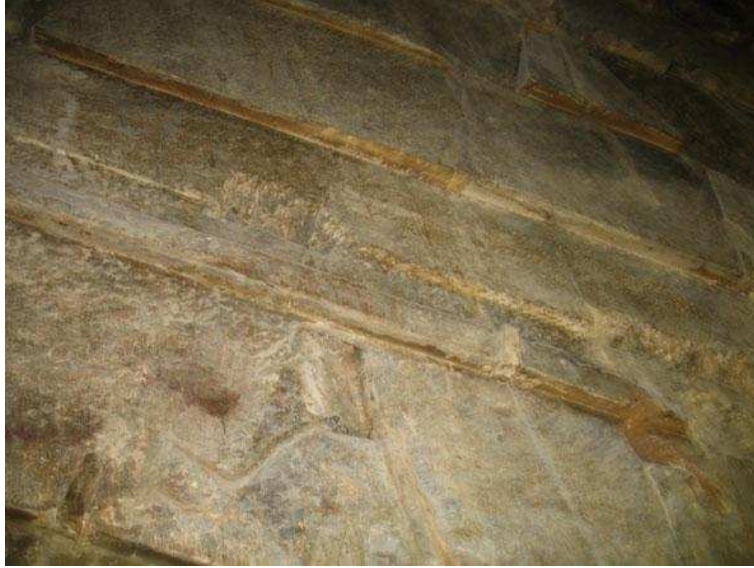
A groove on both sides of the Grand Gallery all along the third corbelling.
