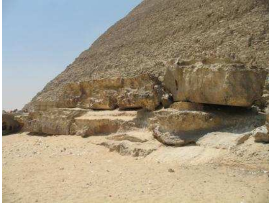
The present platform is made of 2 to 3 layers of huge blocks
