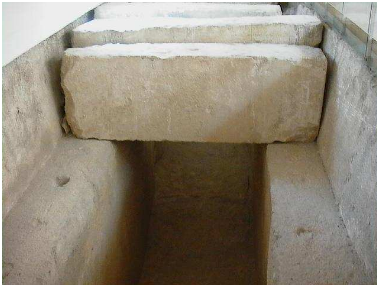
The roofing technique of the Grand Gallery is slightly different from usual corbelling. Some of the slabs were set in place at a later date (pictured here, the roof of the pit of the Khufu's Solar Boat).
