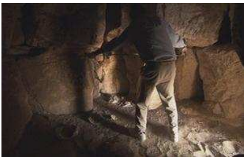
This 3m x 3m room was “built”, meaning that it is a part of the construction, not just a hollow space
