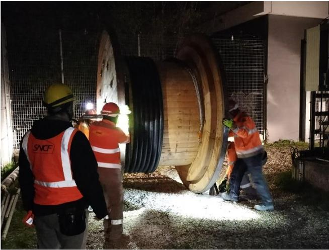
**Fig. 5.** Pulling of a dummy cable in Montparnasse-Vouillé.
