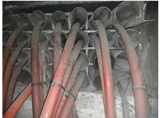
**Fig. 3.** Existing cable duct bank between the substation and the platform. Each conduit is filled with one 400 mm<sup>2</sup> copper cable (500 A each).
