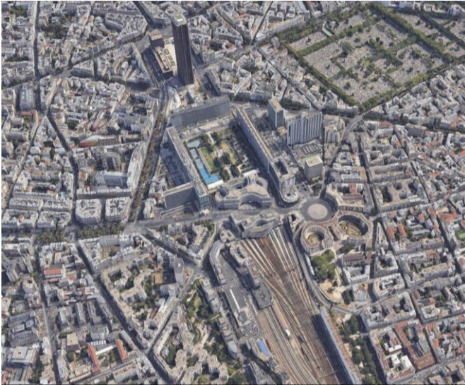
Fig. 1. Montparnasse railway station in Paris, 28 tracks and a daily throughput of 200,000 passengers on 750 trains.
