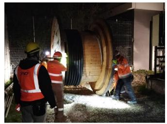
Fig. 5. Pulling of a dummy cable in Montparnasse-Vouillé.
