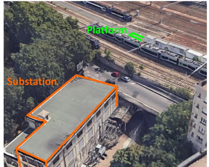
Fig. 2. The Vouillé traction substation (in orange) in the heart of Paris and the railway tracks platform (in green) that will house the HTS cable terminations at Montparnasse station.
