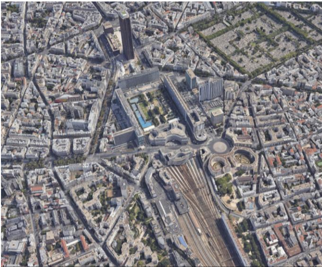
Fig. 1. Montparnasse railway station in Paris, 28 tracks and a daily throughput of 200,000 passengers on 750 trains.
