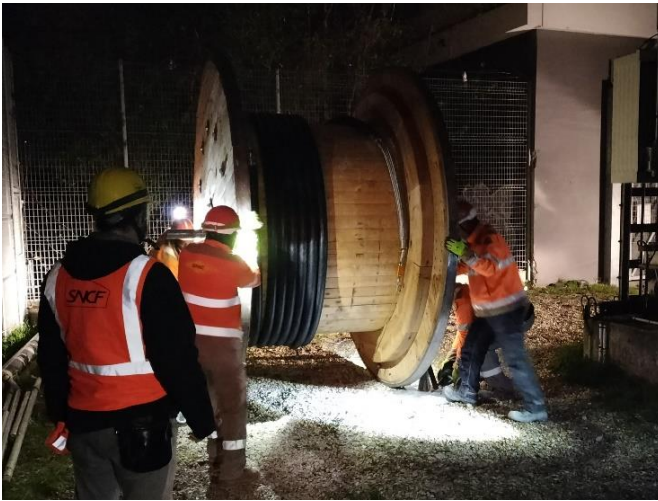
Fig. 5. Pulling of a dummy cable in Montparnasse-Vouillé.
