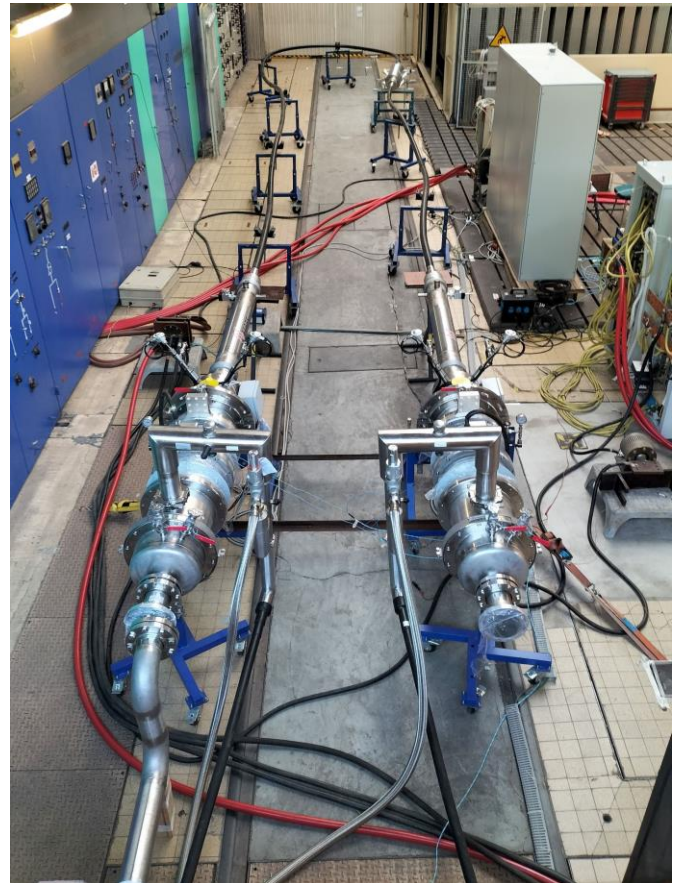
Fig. 12. Cable type test loop installed at the SNCF Railway Test Agency (SNCF-AEF), including two terminations and a joint.
