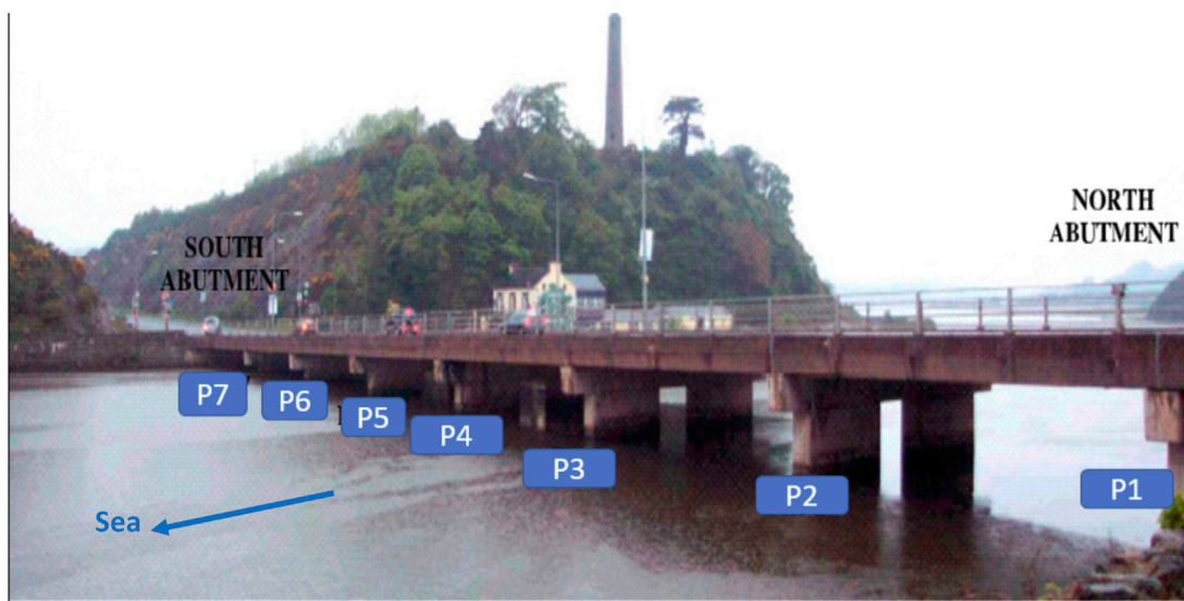
FIGURE 1 Photograph of the Ferrycarrig Bridge (piers #1 to #7 locations) (Kenshel, 2009, pp. 116).
