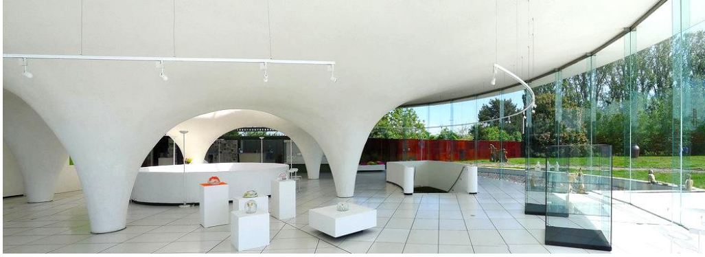
Figure 6: The concrete shell of the Keramion museum in Frechen, Germany, is a Pelikan surface – a special type of i-LW surface also referred to as i-minimal. ©Klaas Vermaas
