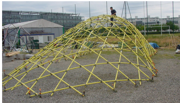
Figure 1: View of the uncovered elastic gridshell.
