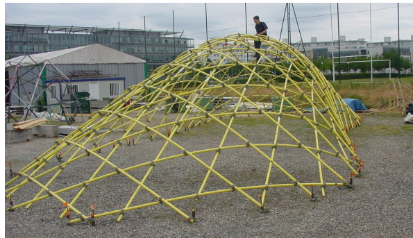
Figure 1: View of the uncovered elastic gridshell.
