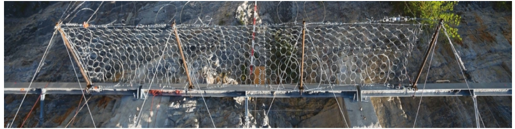
Figure 1. Top view of the experimental set-up (by courtesy NGE fondations).
