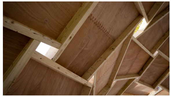
Fig. 8 Bottom of the pavilion. The bottom surface of beams is milled to mask offset and avoid exposure of the timber fibres (credit: Tristan Gobin).
