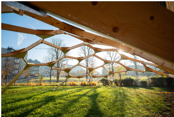
Fig. 21 Timber pavilion with simple beams and complex connectors.
