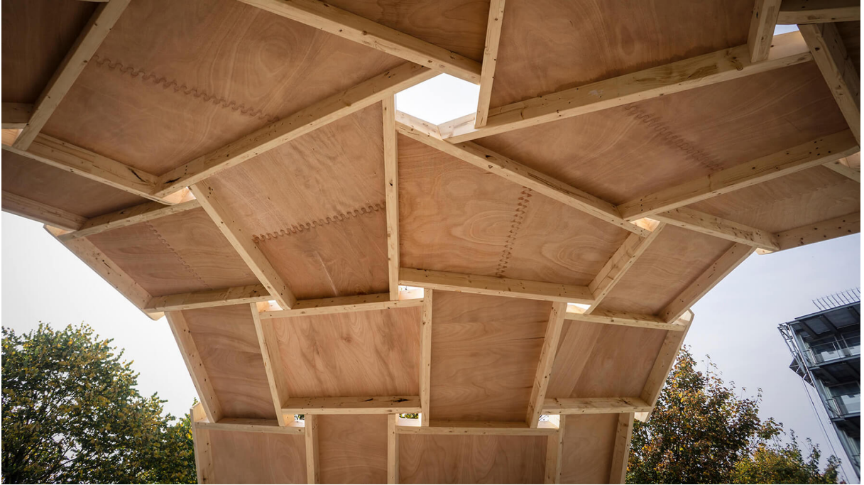
Fig. 5 The shell-nexorade hybrid structure constructed (credit: Tristan Gobin).
