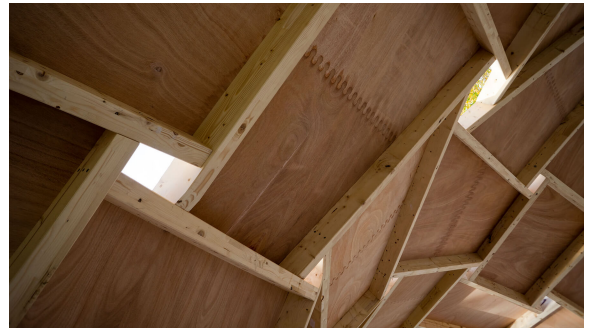
Fig. 8 Bottom of the pavilion. The bottom surface of beams is milled to mask offset and avoid exposure of the timber fibres (credit: Tristan Gobin).
