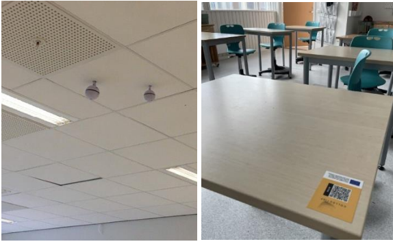
Fig. 7. Picture of the installed IEQ monitoring system and Post Occupancy Evaluation QR code in one of the pilot buildings in Norway
