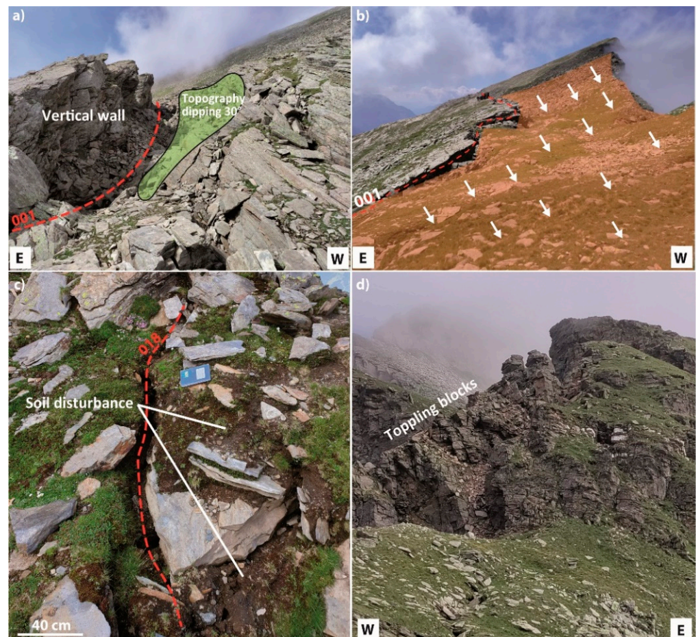
Figure 3. Photos depicting the main characteristics of the Cima del Simano instabilities. (a,b) Main open fracture; (c) Traces of movements in one of the openings near the crest; (d) Fractured blocks in toppling. Their location is shown in Figure 1c.
