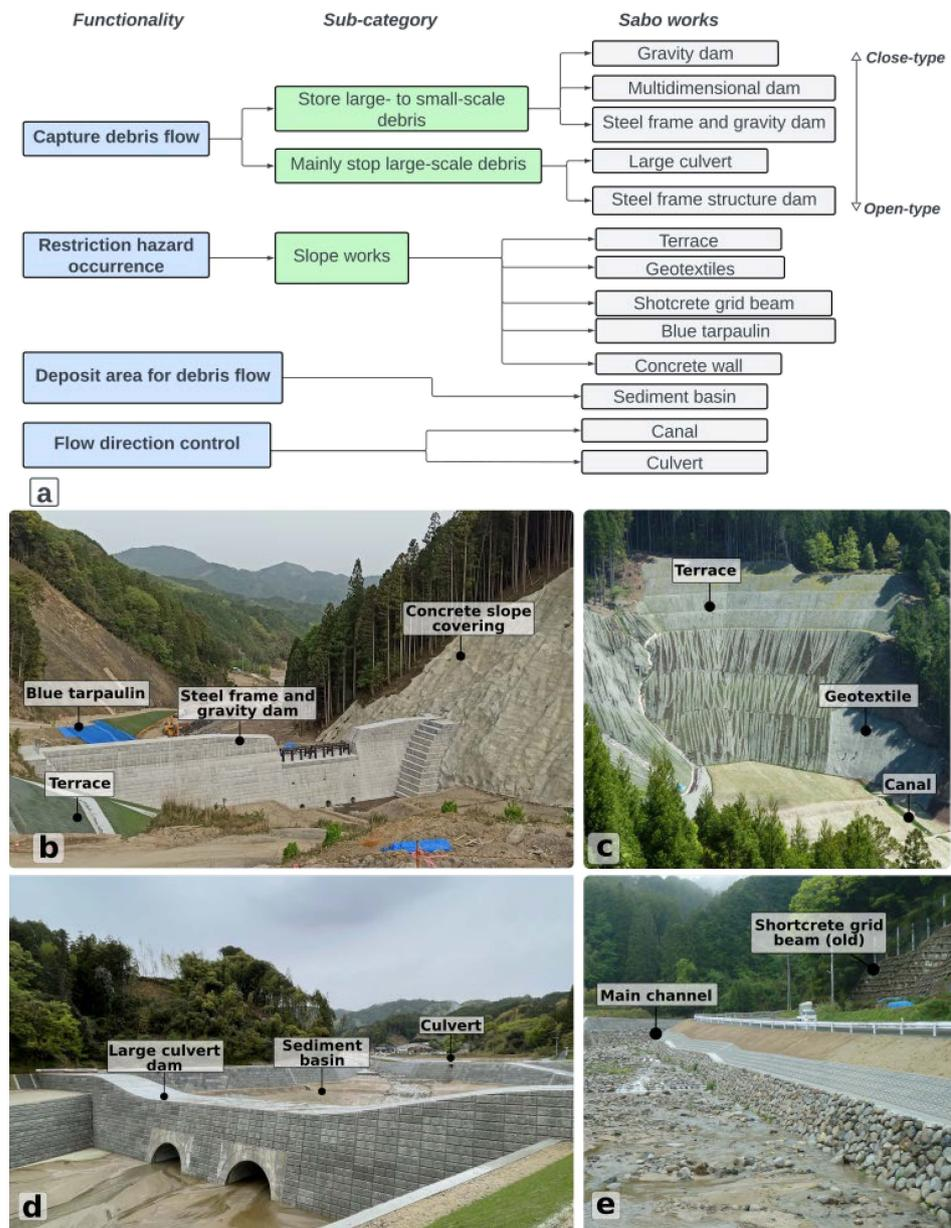
**Figure 12.** (a). Typology of Sabo works in the Otoishi watershed. (b). Area of Sabo dam #15-4 (© M. Dumont, 2023). (c). Reconstruction of slope upstream of Otoishi River (© M. Dumont, 2023). (d). Area of the sediment basin (© G. Arnaud-Fassetta, 2023). (e). Otoishi River channel downstream (© M. Dumont, 2023).
