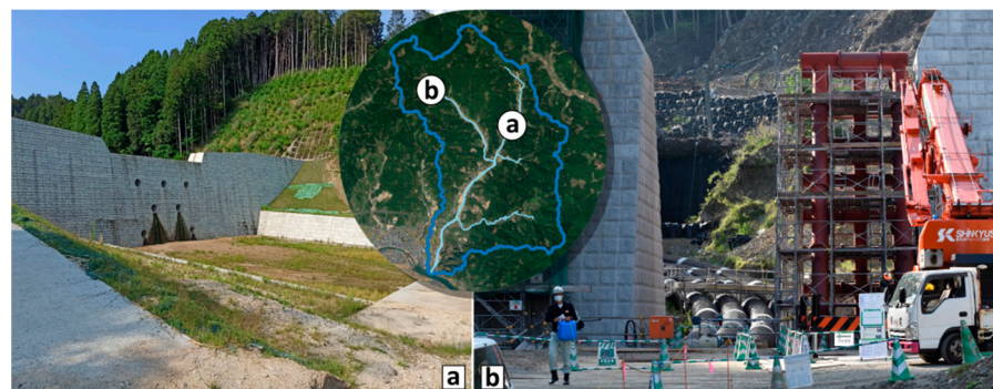
Figure 7. Illustration of the sabo dam constructed in the AK River. (a) Closed-type sabo dam AK16, ©M. Dumont, 2022; (b) slit-type sabo dam OT15-6, ©V. Siccard, 2022.
