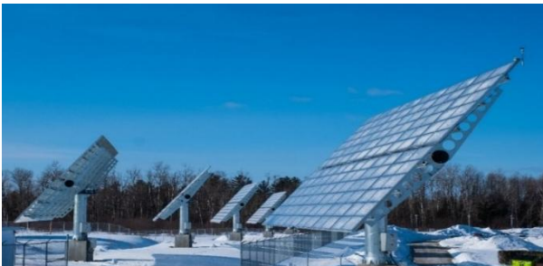
Fig. 2. Five out of eight CPV systems in Université de Sherbrooke solar park, Quebec
