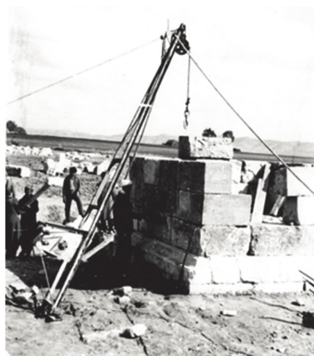
Fig. 4) Mausoleum under works of reassemble in 1967 (Vérité 1988)
