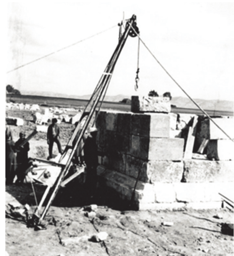
Fig. 4) Mausoleum under works of reassemble in 1967 (Vérité 1988)
