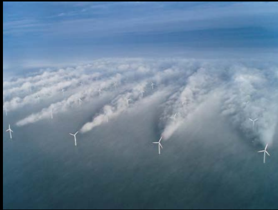
Wake interactions in Horns Rev Offshore Wind Farm
