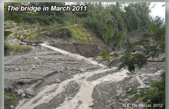
One can notice the ~5m thick deposits accumulated upstream this sabo dam and bridge.
