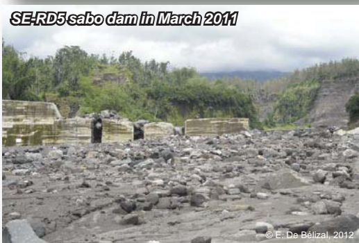
One can notice the ~5m thick deposits accumulated upstream this sabo dam and bridge.
