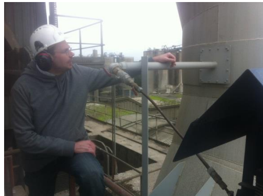
Sampling line connected to chimney stack
