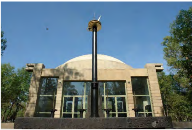
Figure 7. Outside view of Cámara Lambda installed in the back of Cárcamo de Dolores.
