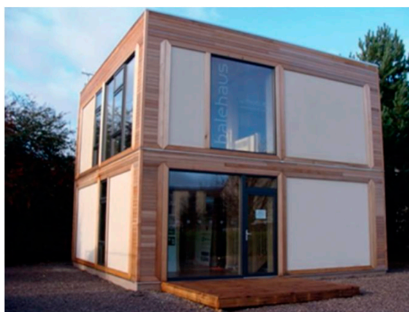
Figure 4. BaleHaus, University of Bath: Straw load-bearing walls [43].
