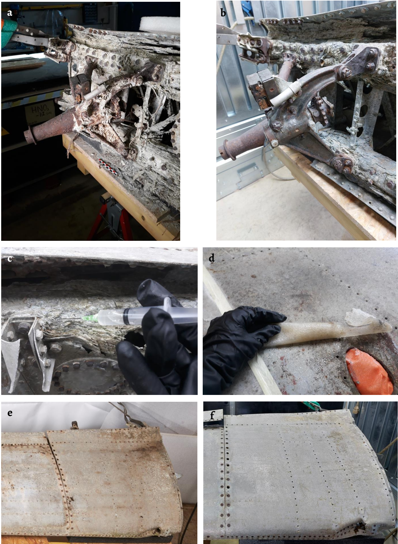
Figure 7. Mechanical cleaning: a) before; b) after treatment; c) consolidation; and chemical cleaning with TAC 5 % w/v applied with Agar gel to 3 % w/v by spray: d) removal of the gel; e) surface before cleaning; f) surface after cleaning.
