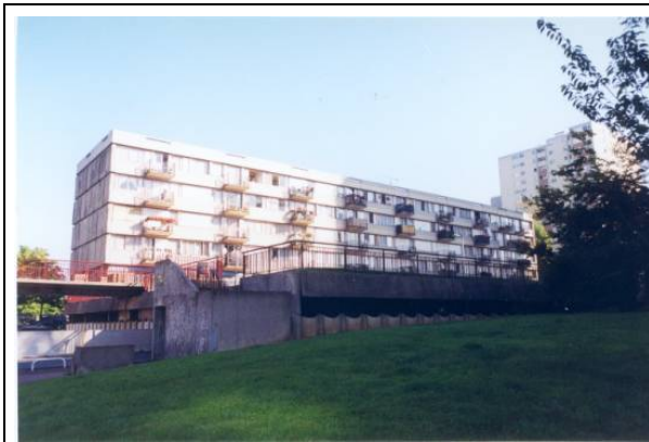
Building before renovation (2000)
