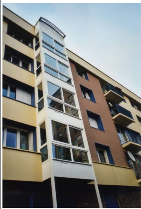
Renovation of the glazed balconies (December 2002)
