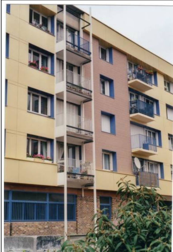
Renovation of the glazed balconies (July 2002)
