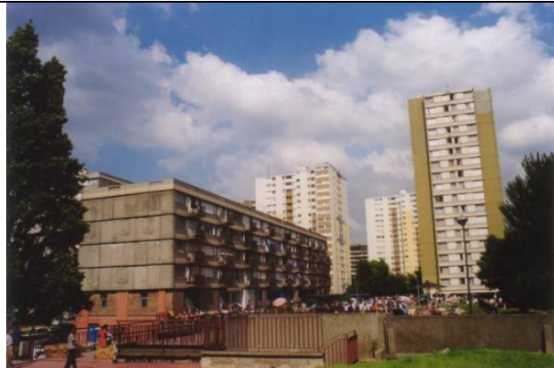
REGEN LINK building before renovation (left)
