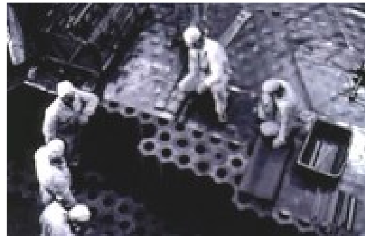
Graphite stack of the moderator
