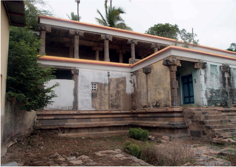
Fig. 6: View from the south-east. The library's pavilion with the new staircase and (to the left) the extension of the library in the gallery.
