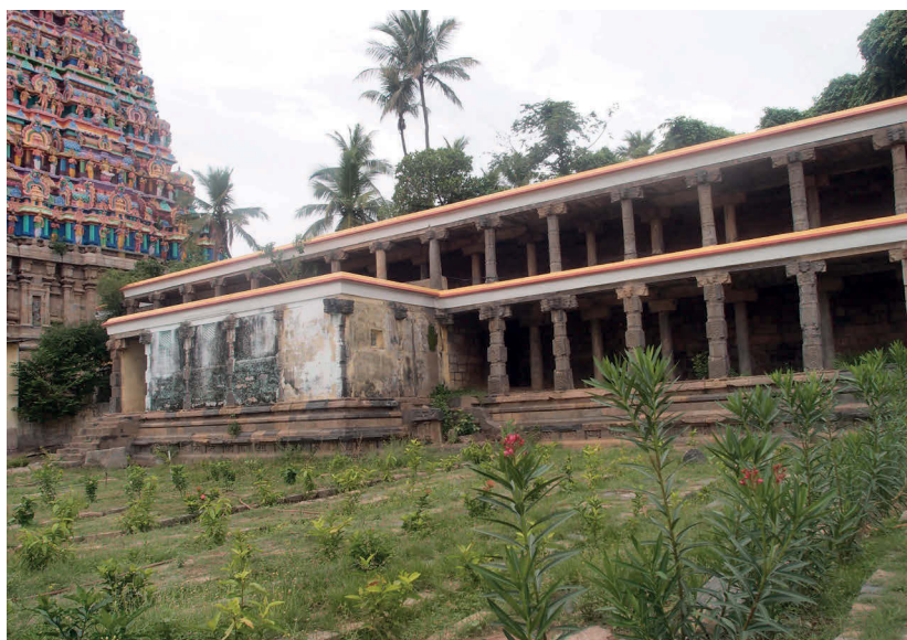
Fig. 4b: View from the north-east: the gallery where the library is located and adjoined with its projecting pavilion (old staircase on the right (north) side) and the garden around.
