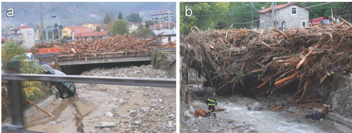
Figure 1: Woody debris accumulations upstream bridges in close vicinity to elements at risk (Lucia et al., 2015).
