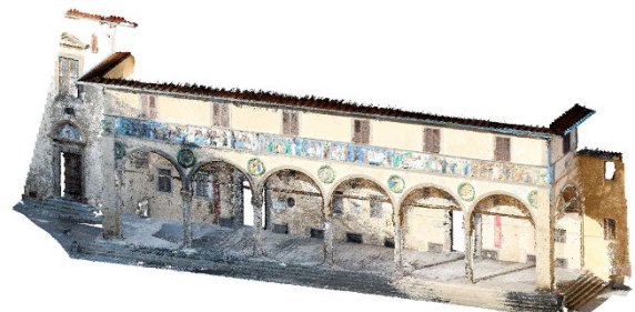
Figure 1. Photogrammetric point cloud of Spedale del Ceppo, Pistoia, Italy.
