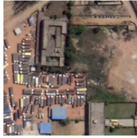
Industrial, Construction Done, Sparse Forest Excavation, Barren Land
