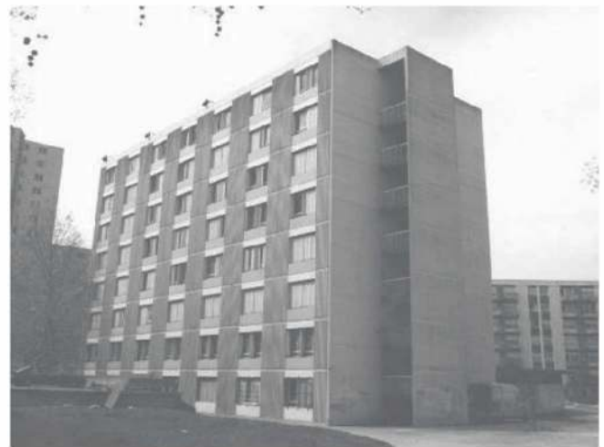
Figure 3. The tested eight-levels building (1970). Height: 22 m. Length: 30 m. Width: 14 m.
