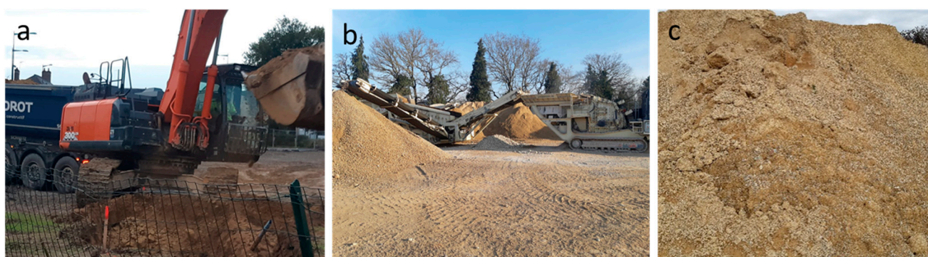
Figure 1. Soil excavation (a), crushing and sieving (b), stockage (c).
