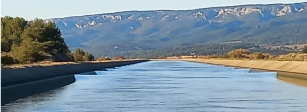
(A) Undular bore in the hydropower canal of Mallemort (France), looking at the incoming bore (Photo EDF)
